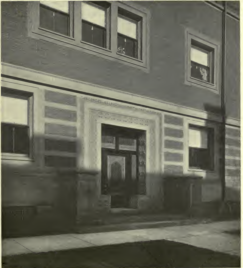
FIG. 3.—ENTRANCE TO THE MADLENER HOUSE.
